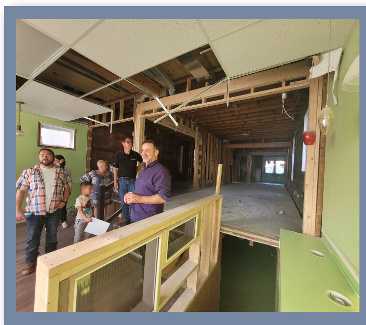
2022 Social Impact Project Tour - Reside Project in construction stage
